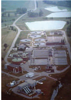
The West Hickman Wastewater Treatment Plant is classified as a two-staged activated sludge nitrification system that treats billions of gallons of wastewater annually.
